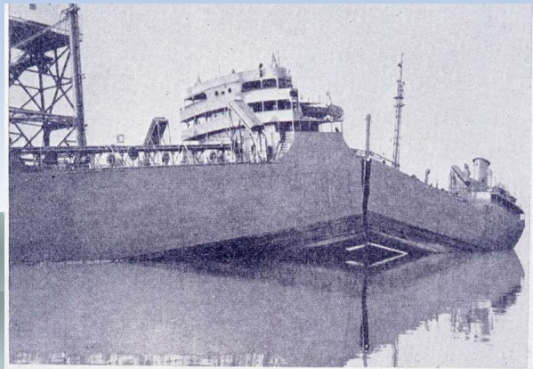
FIG. 1.—The Tanker Schenectady After Splitting in Two at Her Outfitting Dock (1).
